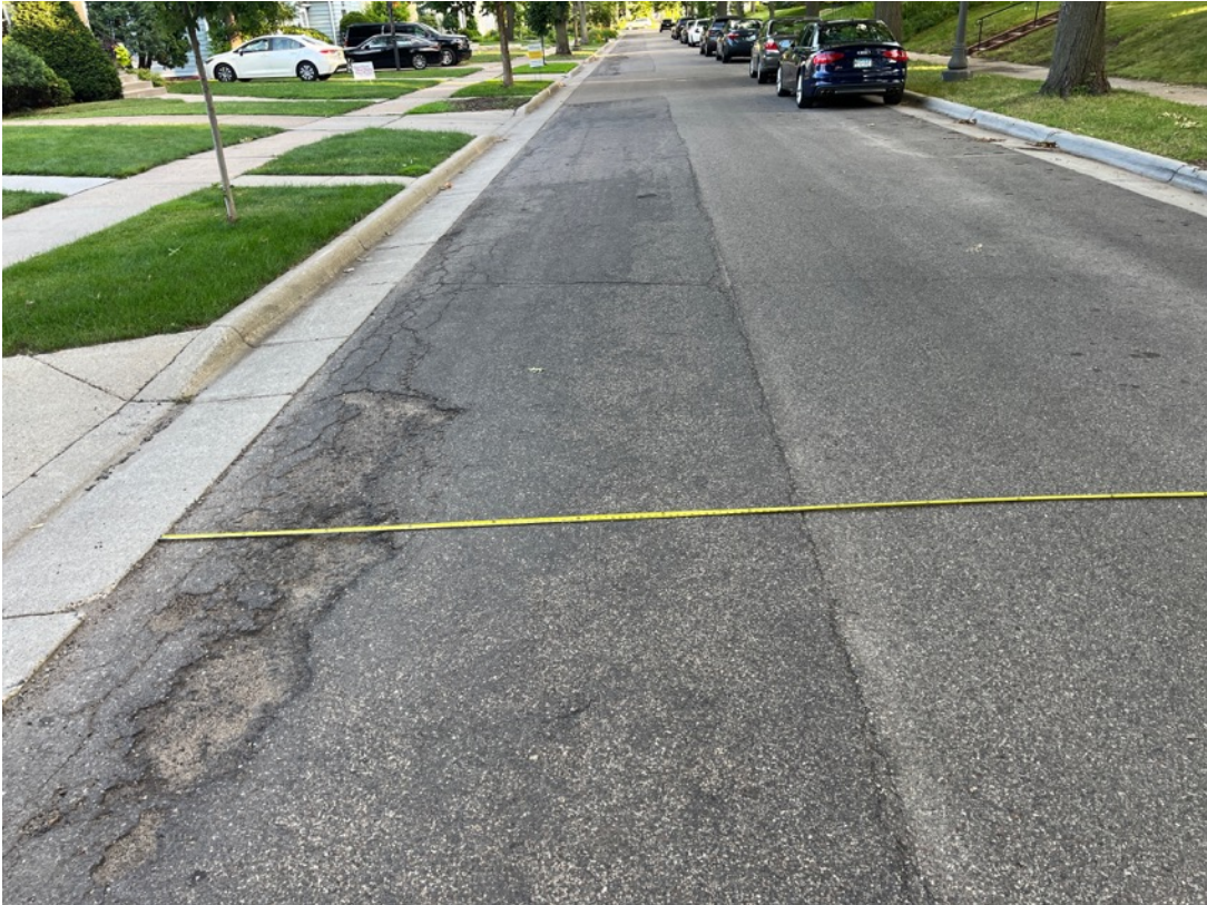
1) View looking south at unreconstructed east lane of pavement (the driving lane), which is full of potholes. Full-width reconstruction is visible at each manhole.
