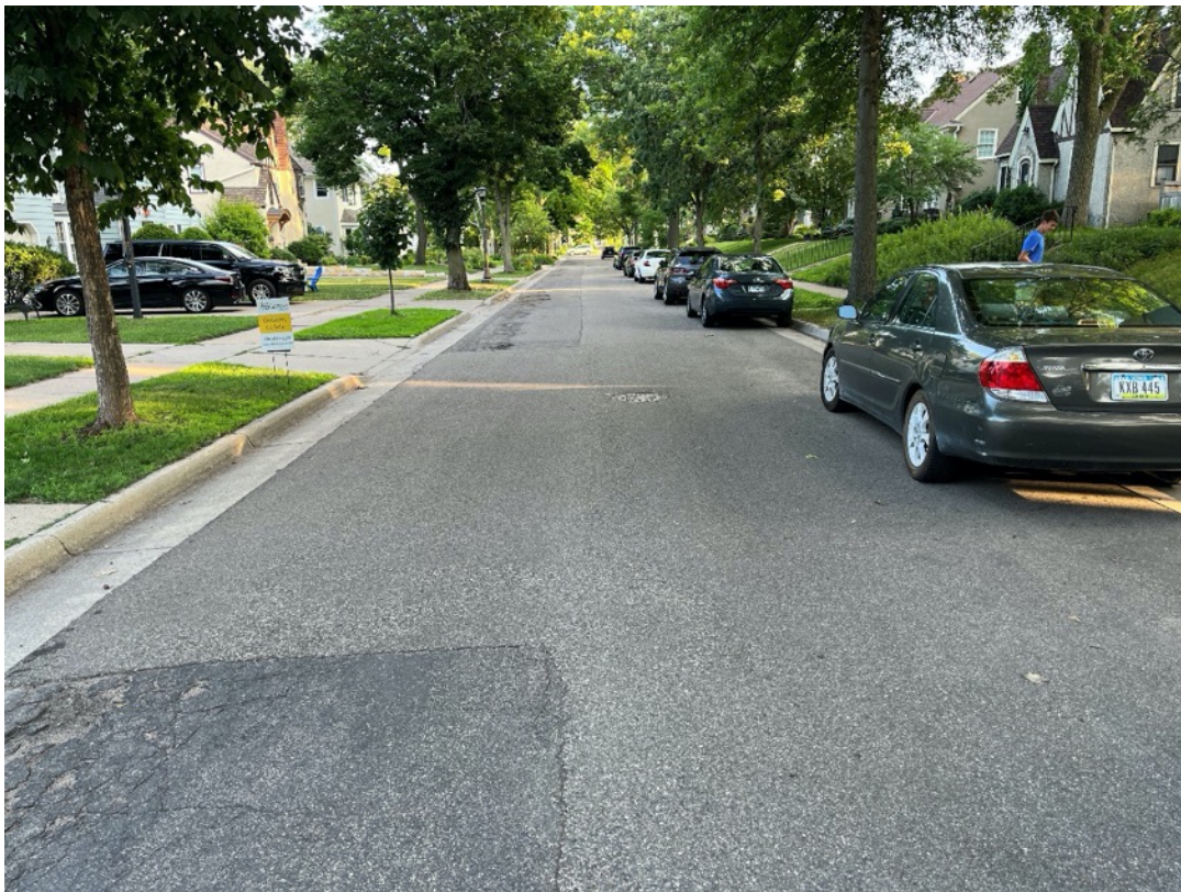
2) View looking south at fully reconstructed pavement around manhole in excellent condition, preceded and followed by unreconstructed pavement in poor condition.
