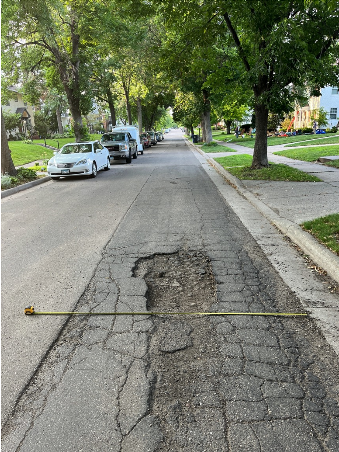
3) View looking north at unreconstructed east lane of pavement (the driving lane due to parking restrictions), which is full of potholes. Full-width reconstruction is visible at each manhole.
